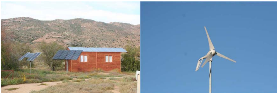
Solar system and wind turbine at the research station.
